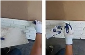
6.FILLING SEAMS, TRIMMING EDGES, CLEANING
